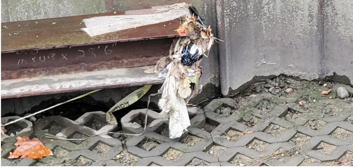
Trash caught on steel bracing for retaining wall.
