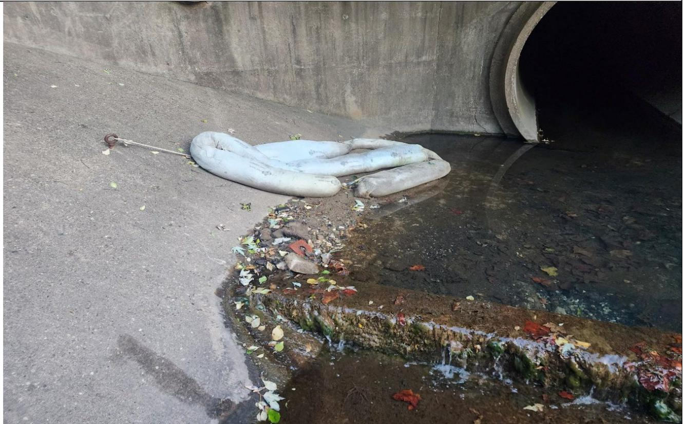
Sediment sock has broken loose from its second anchorage point and was moved to the side.
