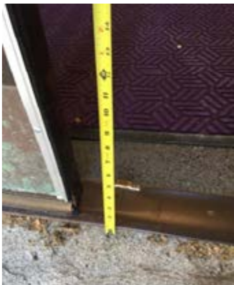
Figure 18- High Threshold
