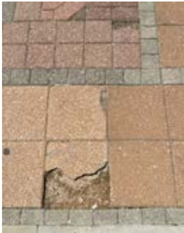
Figure 12- Cracked Panel
