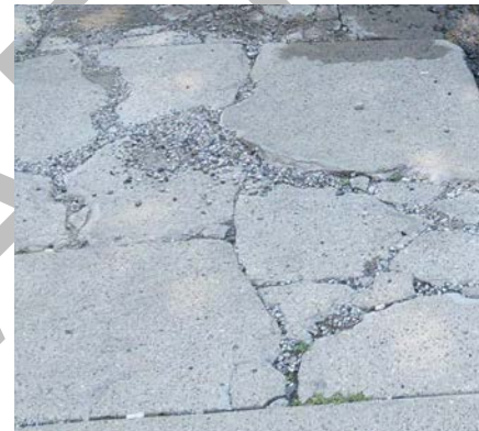
Surface Condition: Cracking
