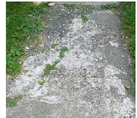
Surface Condition: Spalling
