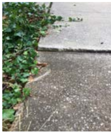
Figure 13- Vertical Fault
