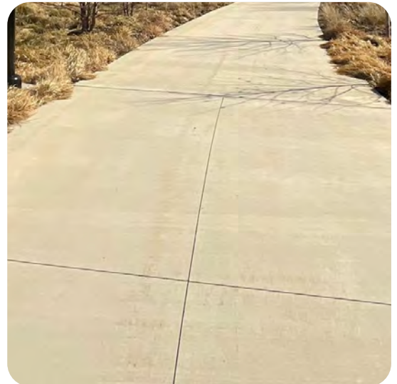
Primary walkway concrete application with standard jointing pattern in the Military Axis
