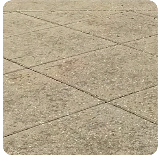
Primary walkway concrete application with 45-degree jointing pattern on the Main Quad
