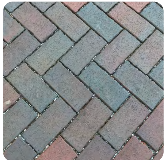
Clay permeable paver application on a secondary walkway
