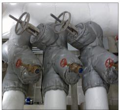
Overheating in mechanical spaces costs the campus in lost energy efficiency. The heat/frost insulators add recyclable insulating materials to pipes and equipment, providing energy conservation and burn protection, as well as reducing unnecessary wear and tear on other mechanical room equipment.
