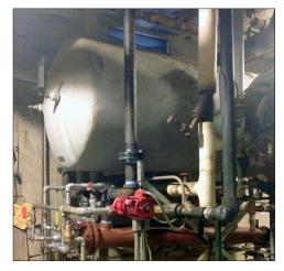
The heat/frost insulators prevent loss of mechanical heating and cooling in HVAC systems.
