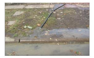
The Illinois Environmental Protection Agency (IEPA) regulates storm water dewatering activities to storm sewers by requiring sediment control and inspections for dewatering activities. These guidelines are designed to protect waterways by preventing or minimizing sedimentation.
