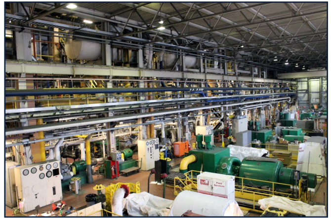
Abbott Power Plant
