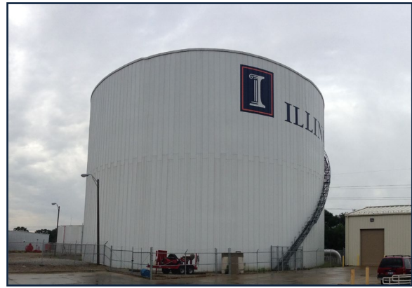
Thermal Energy Storage Tank
