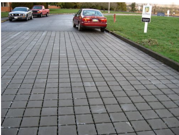
Figure 3. Pervious pavers used in the roadway of a neighborhood development in Wilsonville, OR
